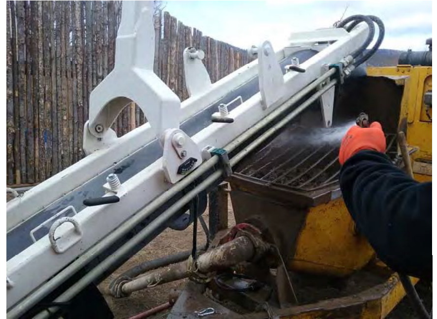
PHOTOGRAPH 22: Mixing grout
