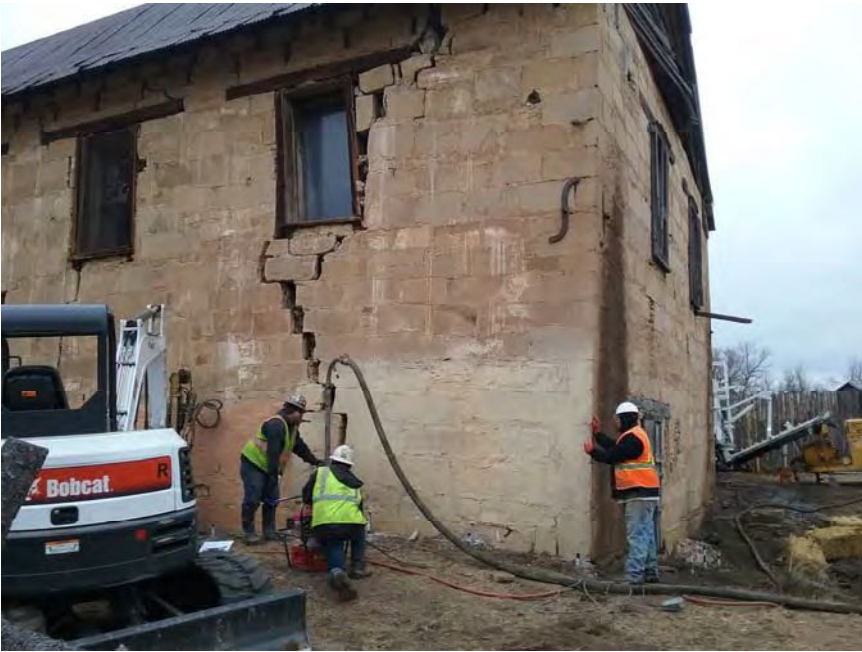
PHOTOGRAPH 23: Pumping grout at East wall crack
