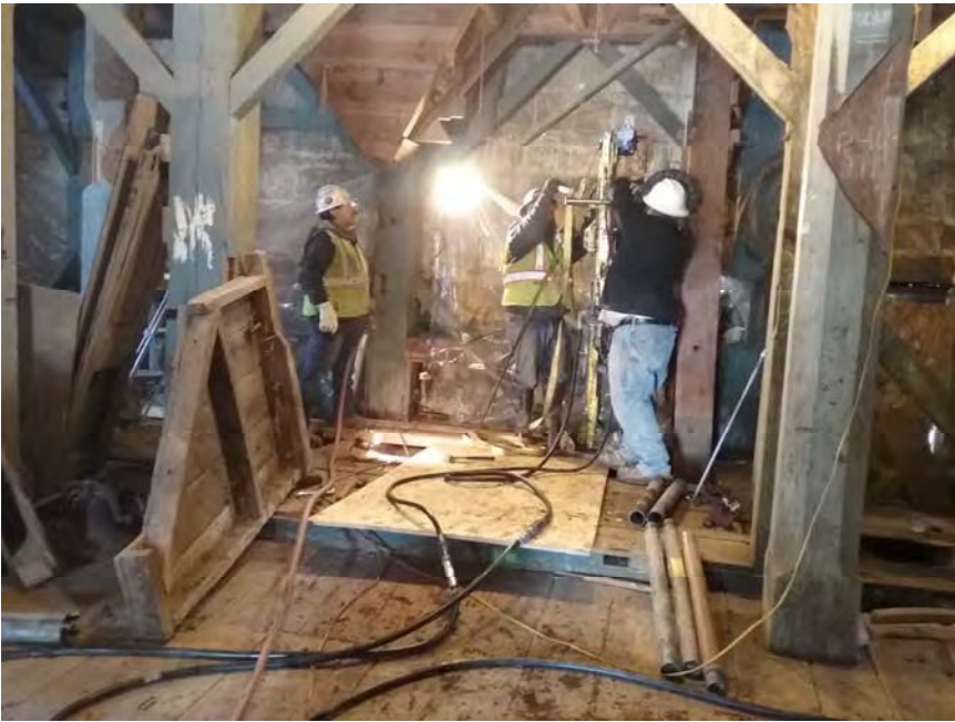
PHOTOGRAPH 27: Drilling inside N. wall
