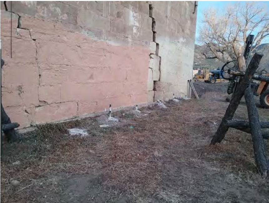
PHOTOGRAPH 5: East wall permeation grout locations
