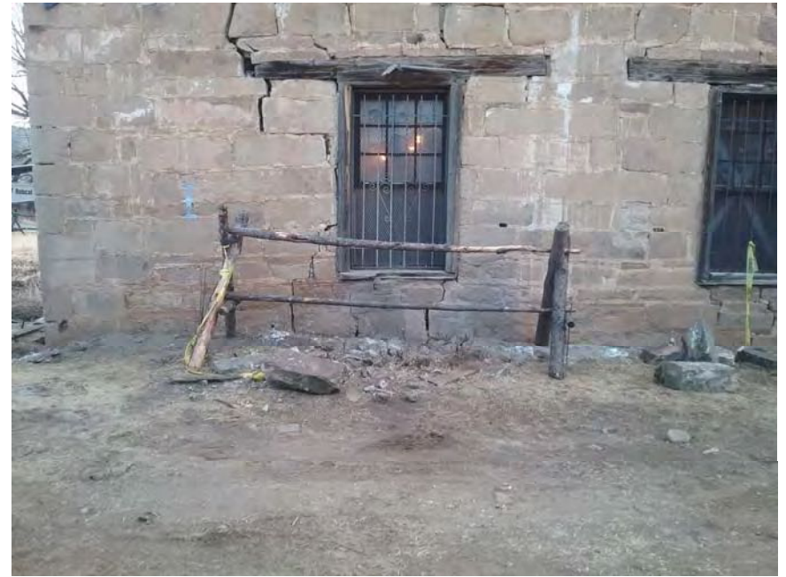
PHOTOGRAPH 4: West wall falling rock
