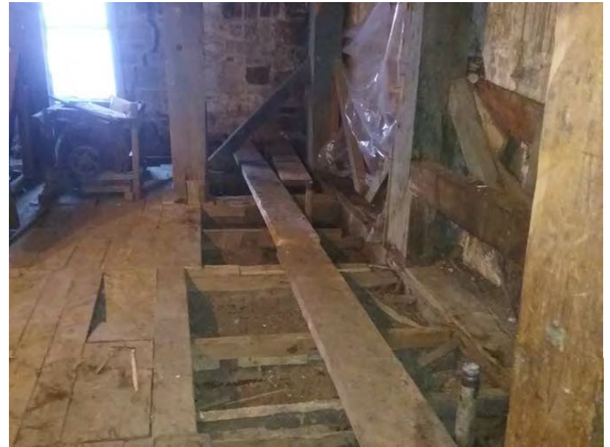
PHOTOGRAPH 30: Removed floor planks inside N. wall
