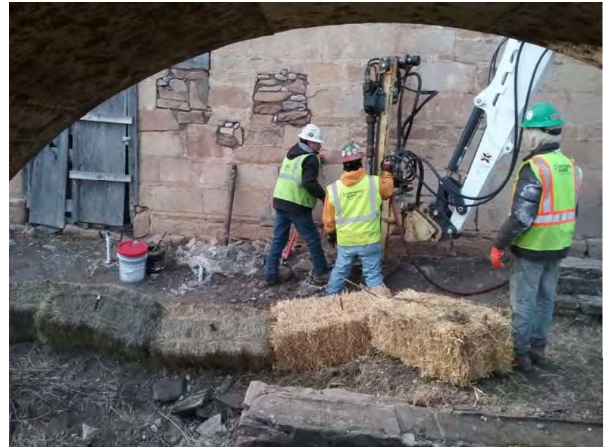
PHOTOGRAPH 14: Drilling at N. wall with mini-excavator
