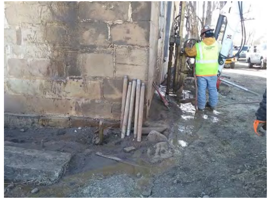
PHOTOGRAPH 20: Drilling at N.W. corner (west wall)
