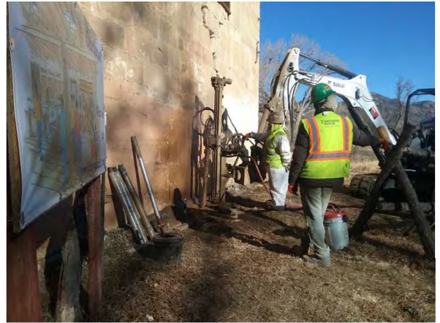
PHOTOGRAPH 28: Drilling full depth outside E. wall
