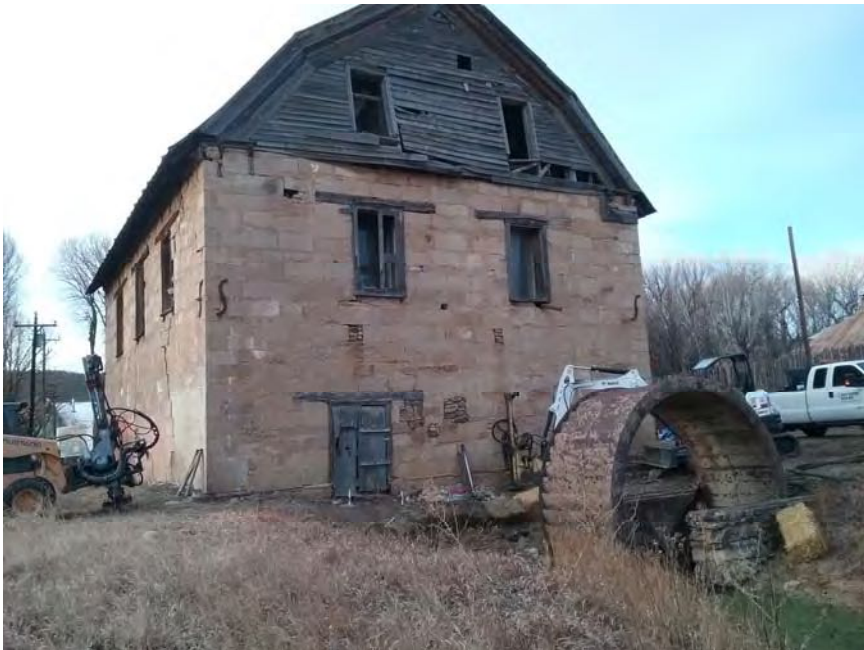
PHOTOGRAPH 11: Water wheel N. of building
