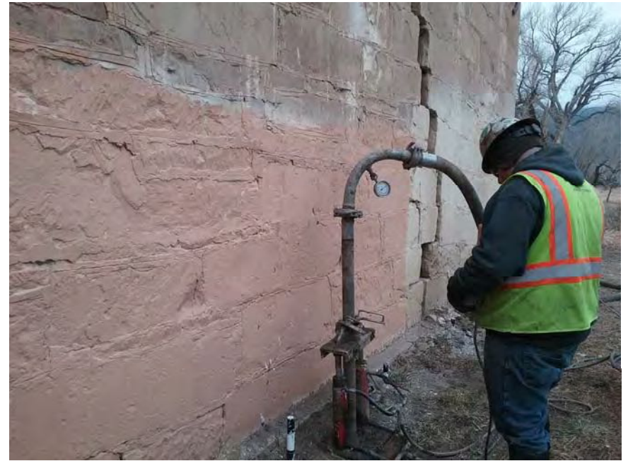
PHOTOGRAPH 24: Pumping grout outside E. wall
