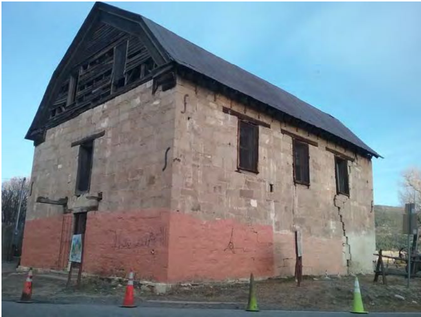
PHOTOGRAPH 1: Mill looking N.W.
