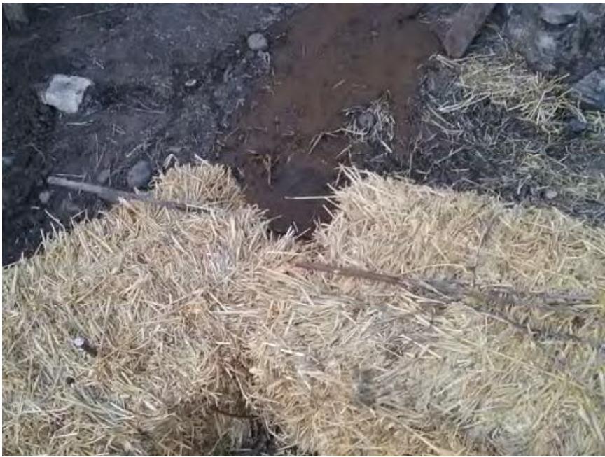
PHOTOGRAPH 19: Drilling water at straw bales
