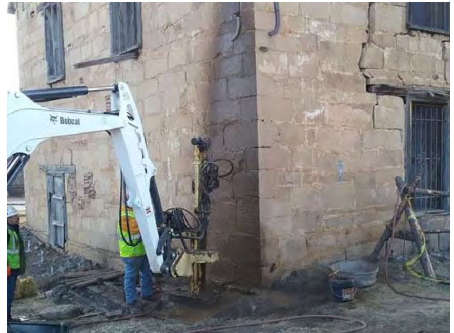
PHOTOGRAPH 18: Drilling at N.W. corner (north wall)
