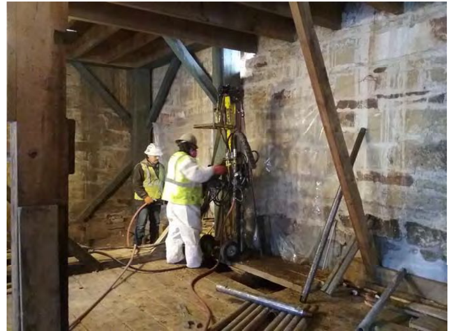
PHOTOGRAPH 26: Drilling inside E. wall
