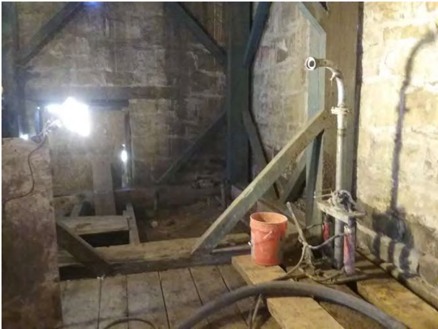
PHOTOGRAPH 29: Grout pumping setup inside E. wall
