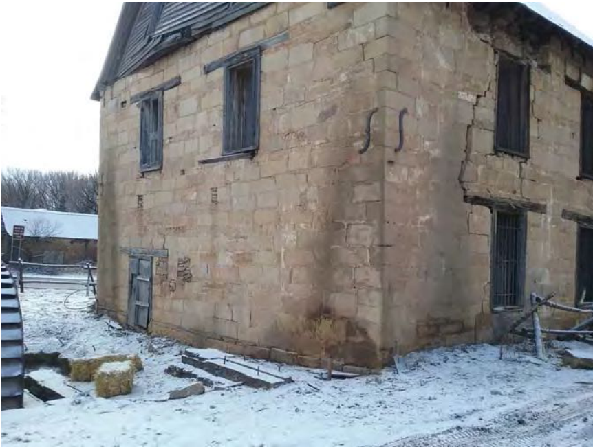
PHOTOGRAPH 25: N.W. corner after snow (looking S.E.)
