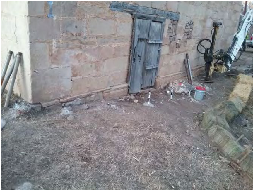
PHOTOGRAPH 9: North wall permeation grouting
